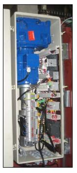
The CONDOR is a compact door which means that the drive unit, consisting of a geared motor for normal supply, a 24VDC motor (for emergency drive above bulkhead), electrical control plate and push
